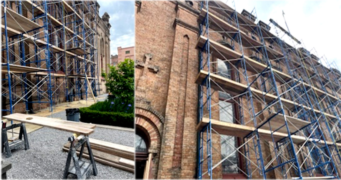
PHASE I - EXTERIOR Restorations are underway
