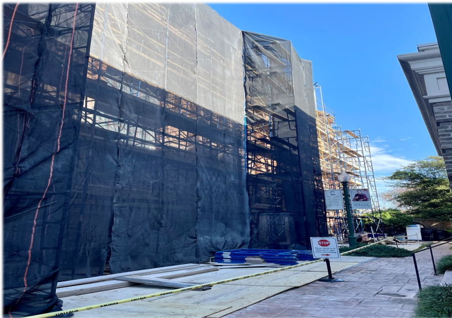
PHASE I - EXTERIOR Renovations are underway (on the riverside of the Church) (picture taken: Dec. 14, 2024)
