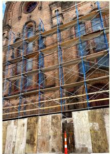
Save St. Mary's Restoration/Phase 1 Project Update: The exterior restoration and repairs have just wrapped up on the riverside of the church. You will notice that scaffolding has gone up in front of the church, on Josephine Street and the contractors will continue removing old mortar and replacing bricks, and all exterior repairs as needed. We appreciate your prayers and support of this project.
