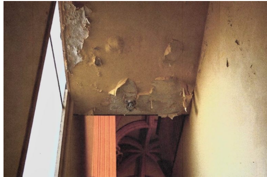
Some pictures of the interior damage and repairs needed to the church's ceilings, walls, plaster moldings and decorations, and repainting restoration.
